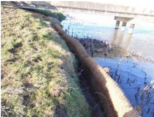
Additional flood risk activity within the Catchment Action Plan includes reducing bank erosion through 'toe protection work' e.g. using coir rolls shown here.
